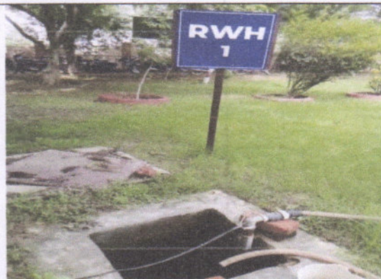
Fig 17. Rainwater harvesting recharge pit
